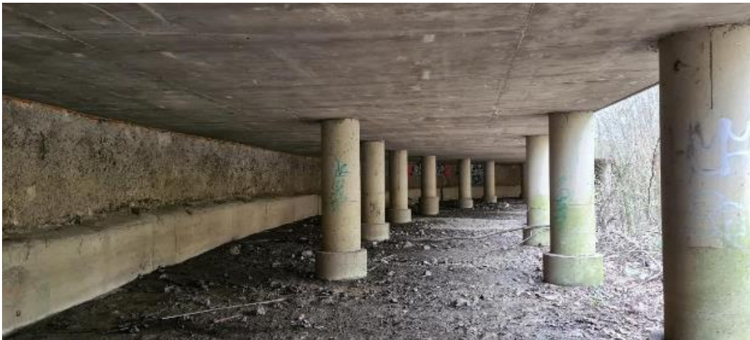
Figure 14: View from the stilt structure supporting Longbridge SLTL
