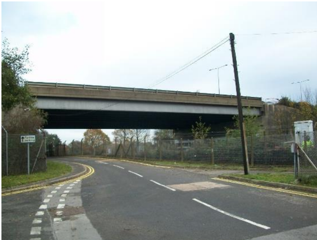
Figure 24: Existing Airport Way Bridge
